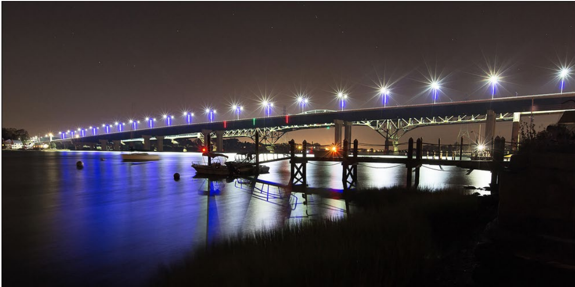
SAKONNET RIVER BRIDGE
