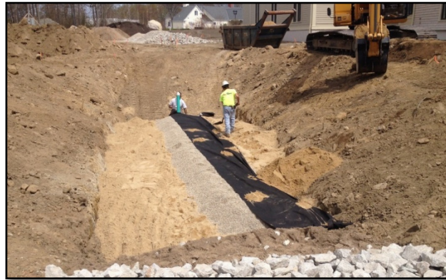
BIO-RETENTION DRAINAGE SYSTEM INSTALLATION
