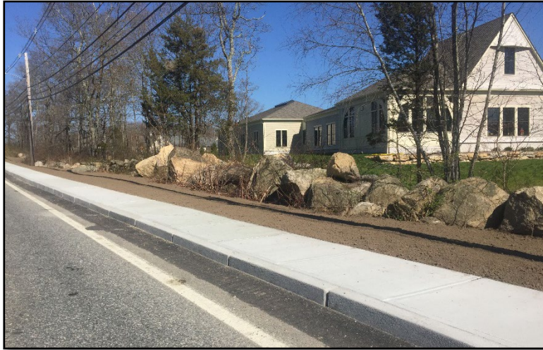
NEW SIDEWALK ALONG BULGARMARSH ROAD
